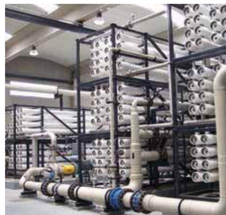
In the Camp de Tarragona Water Reclamation Plant, effluent passes through an enhanced physico-chemical pretreatment process before reaching the reverse osmosis stage. Photo by Veolia Water Solutions & Technologies
