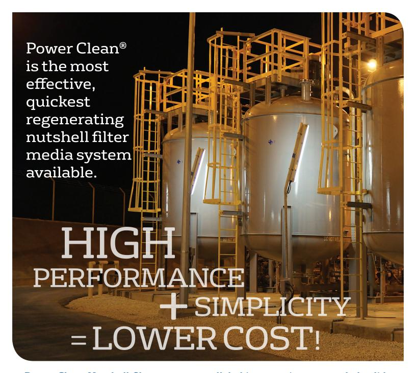
Power Clean Nutshell filters are unparalleled in removing suspended solids and hydrocarbons from produced water or any water source. They are equally effective for the treatment of suspended solids, oily residues, ash and metallic hydroxides from industrial liquids generated by metalworking, power generating, municipal, chemical or petrochemical industries.
