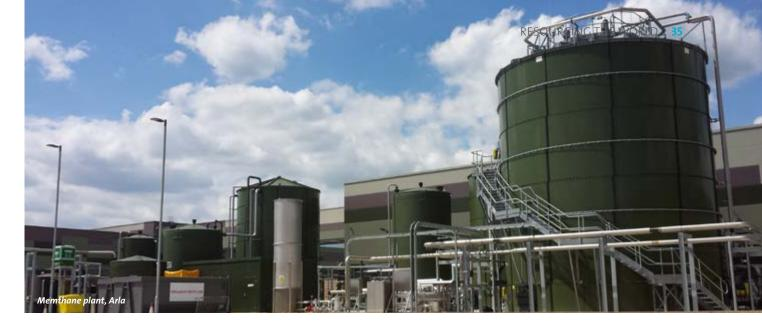
Advanced settlers are installed, which separate the biomass from the final effluent and the biogas. The system is designed for 2,800 m³/day of wastewater and produces more than 9,000 Nm³biogas per day (approx 2.8 MW).
