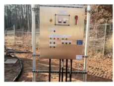
Dedicated control system with Intelligent programmable relay (Zelio) or PLC with HMI. All automatic sequences of operation, manual operation, protections and alarms included. Local control station for tests and maintenance (if applicable). Standard control system and custom system upon client standards are available. Design and engineering by Veolia.
