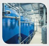
a carbonated »mineral water« of drinking water quality that is free of solids. Unlike other desalination technologies, with **CARIX**<sup>®</sup> there is no salinisation of the wastewater that would otherwise be caused by the regeneration chemicals or the entry of phosphates when using antiscalants (nanofiltration, reverse osmosis).
