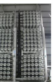
Among the various processes, membrane desalination via reverse osmosis (RO) has become the most widely used solution.
