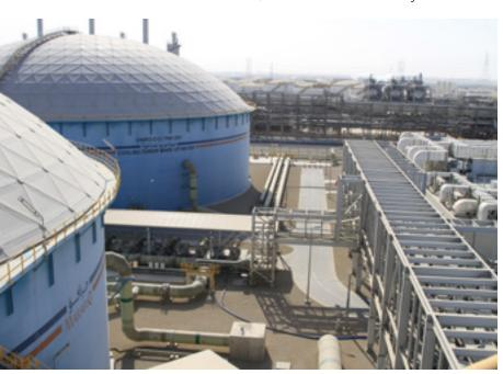
Product water storage tank for cooling tower make-up water.
