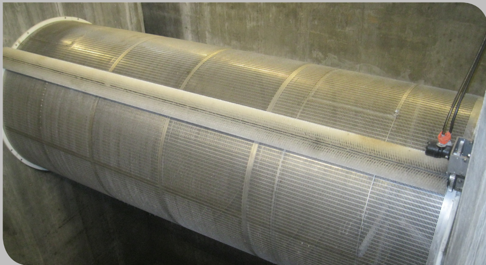
Figure 1: HYDROVEX® RDS Typical Installation
