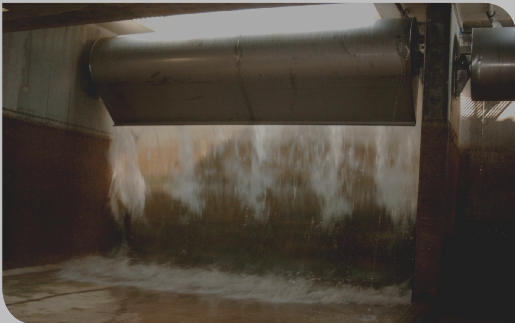
Figure 1: HYDROVEX® SFT Flushing
