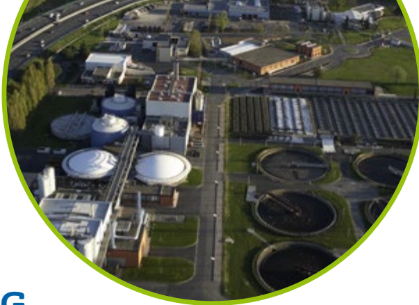
Ginestous-Garonne wastewater treatment plant in Toulouse, France
